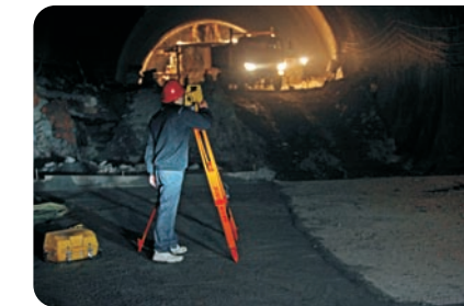
Tunnel Construction Used for drilling and orientation with reliable machine guidance
